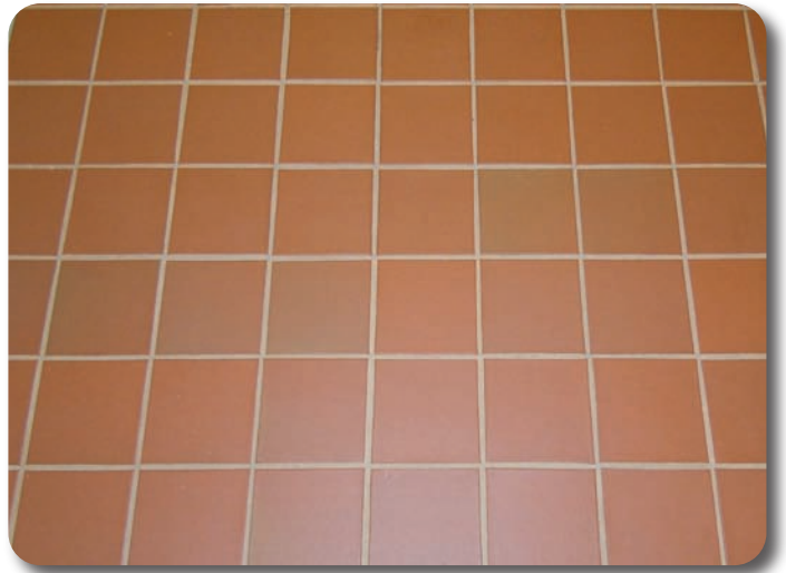
After the Surtec Tile & Grout Restoration
