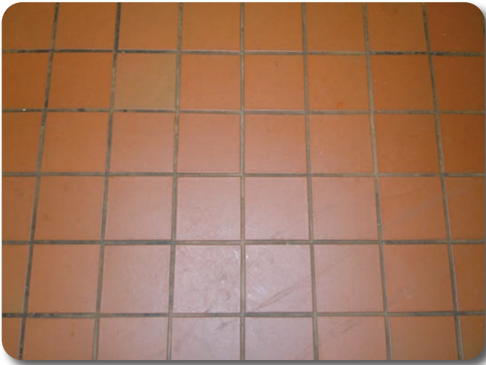
Before the Surtec Tile & Grout Restoration
