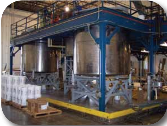
Surtec Chemical Manufacturing Area
